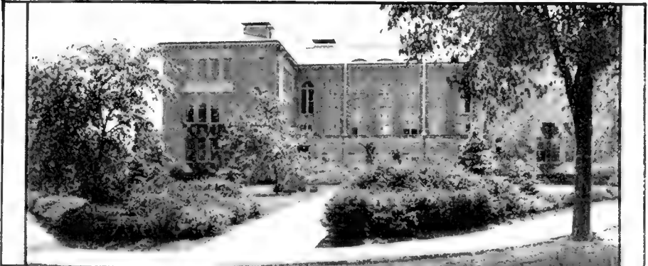
THE RAW BUILDING - WELDED INTO THE LANDSCAPE
